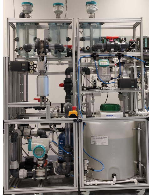
Fig. 6: Experimental setup: The top three tanks correspond to tanks B1, B2, and B3 (from left to right). The black boxes in the middle of the image are the pneumatic valves V1 and V6 (from left to right). At the bottom of the picture are the pump and the reservoir tank B1.
